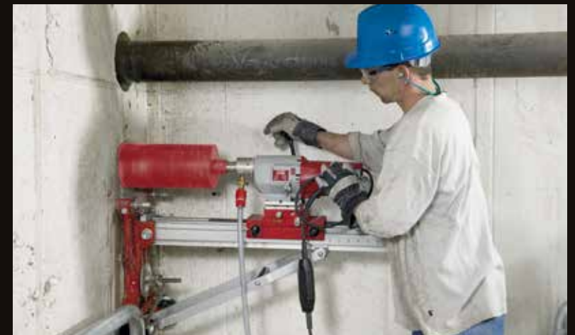
Diamond drilling rig
